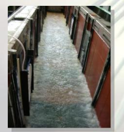
Suction hoods alongside the tank made in polypropylene and complete with setting panels on the suction holes
